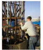
Installation of reinforcing cage with O-cell
